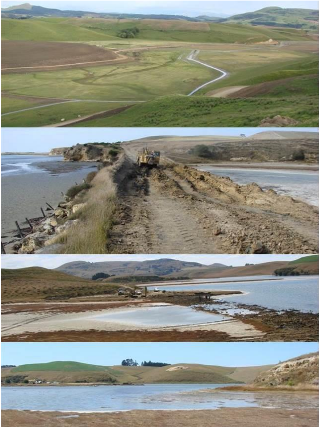
Figure 3: Restoring the tidal flow to the southern arm of the Pleasant River Estuary in 2009. The top photo shows the paddocks in the upper reach of the estuary arm before the causeway was removed. Photos by Irene Walton.
